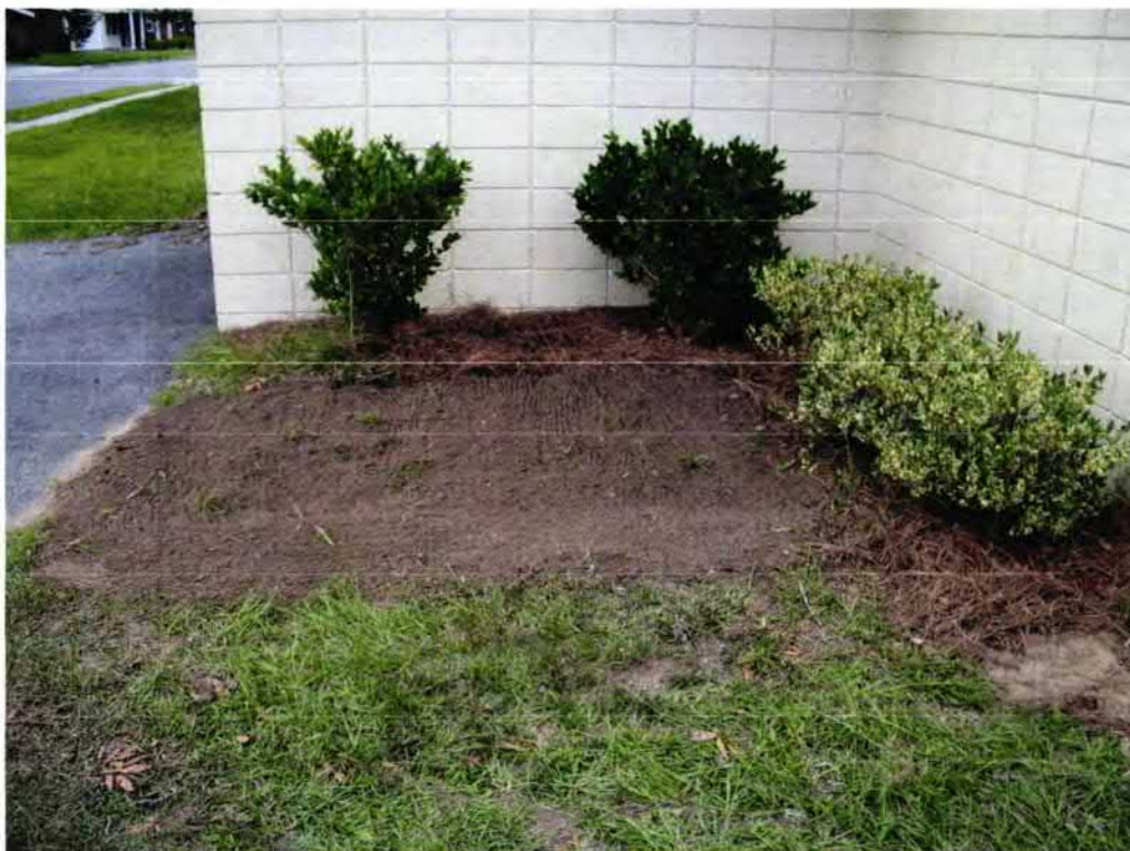
Picture 2: UST 855Dolphin excavation site at job completion.
